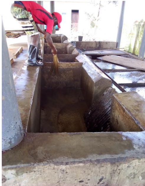
Figure 4-8: Holding facility for non-vacuum sludge discharge
