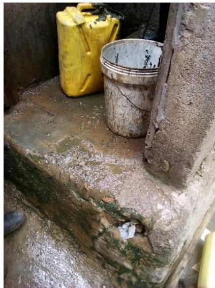
Figure 4-12: Unhygienic manual emptying with sludge spills
